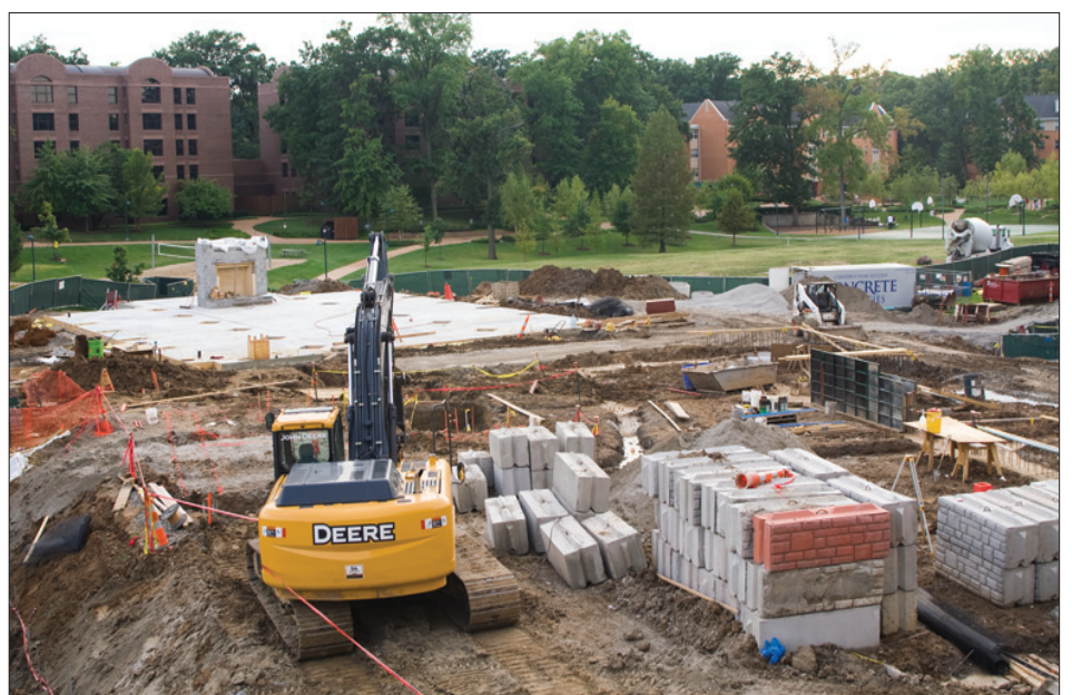
Construction on the South 40 moves into Phase II, which includes College Hall and Eliot B. On Monday, ResLife and Dining Services representatives presented their vision for the South 40 to students.
