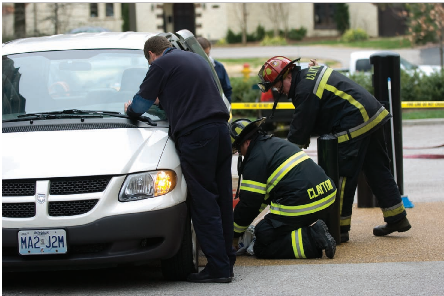
Clayton firefighters work to stop a gas leak Tuesday afternoon on the Danforth Campus. Students could smell the gas from the leak in the air surrounding Brown and McDonnell halls, but the leak didn't affect the insides of the buildings and didn't force any evacuations. According to a University facilities worker, the leak was caused by a ballard puncturing a gas tank under the asphalt.
