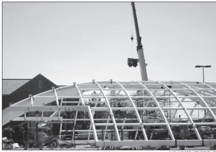
Construction in front of the law school covers the place where a parking lot and pathway to the South 40 and B-school used to be.
